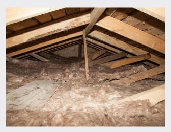
Allowing air to enter a roof space ensures moisture and condensation can move into the atmosphere. If the moisture and condensation has nowhere to go then any moisture can sit on the timbers. This can lead to timber defects such as rot forming and it can also leave the timbers at risk of wood boring insect attacks.
